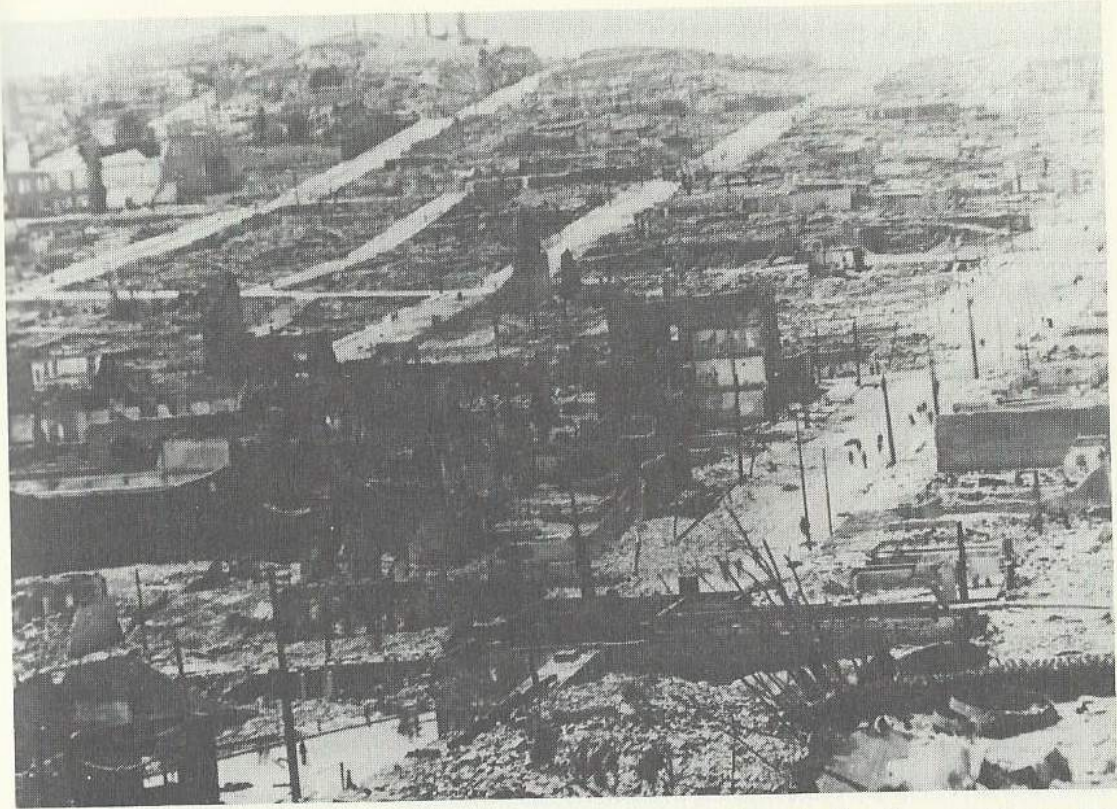
Only a fifth of the total destruction was caused directly by the earthquake; the rest came from the ensuing fire.
